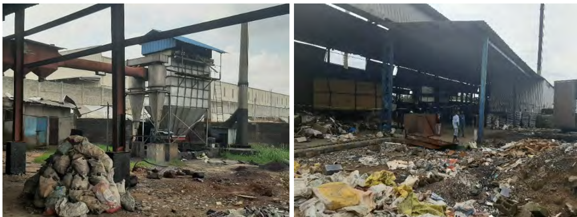
Figure 5. Baghouse at KYSEN recycling plant (left) and partial view of the GANESHA Cameroon Sarl plant (right).
